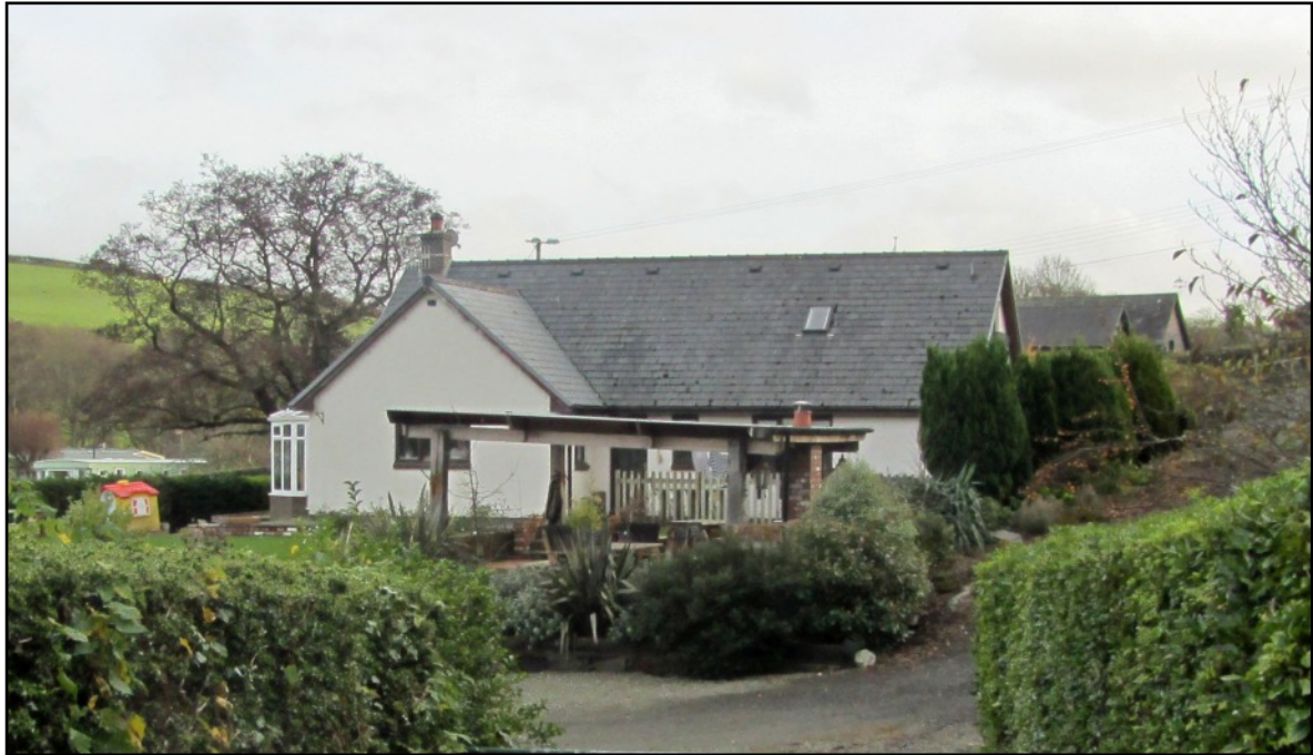
ABOVE The west side of Felinwern in 2015. This has its garden with a loggia. On the right is sloping hillside up to the road.
