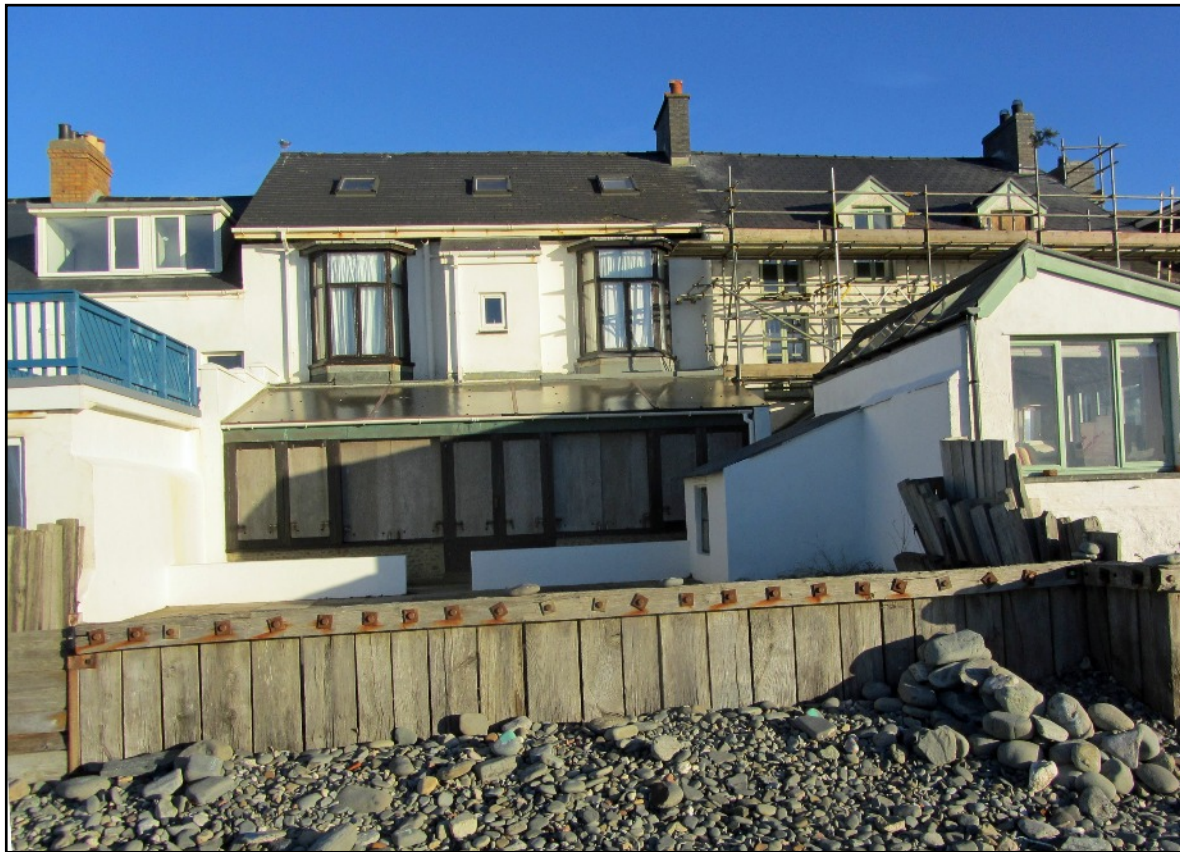
ABOVE The rear of the house in 2016 from the beach. Running along the back of the house is an extension of the ground floor like a sun room, but in this photograph it is protected from the sea in case of a bad storm. There are oriel canted bay windows above it and a small extension in the centre of the back.
