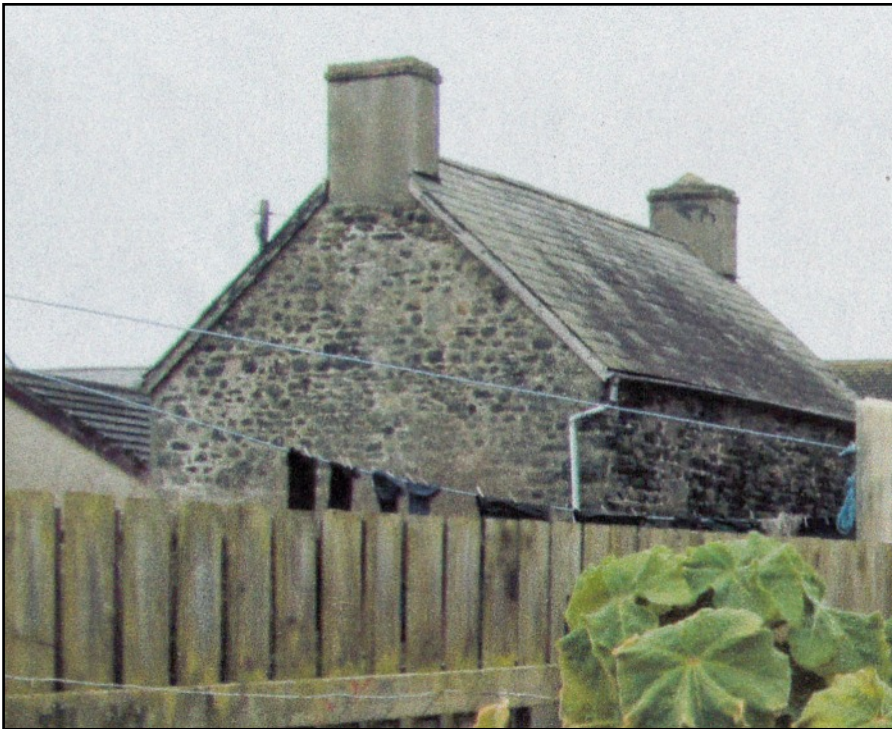
LEFT The north side and east end of The Elms, all rubble stone.
