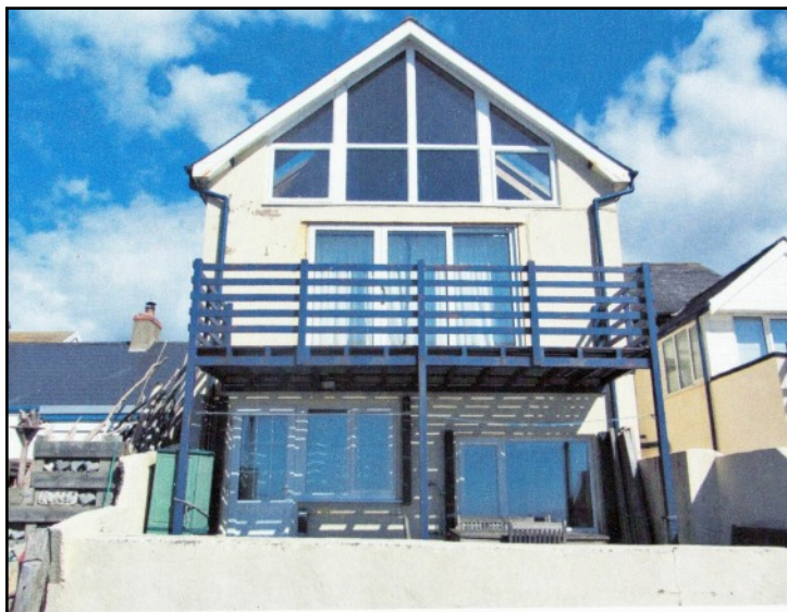
LEFT Deudraeth from the beach in 2015. BELOW LEFT the north face of the extension.
