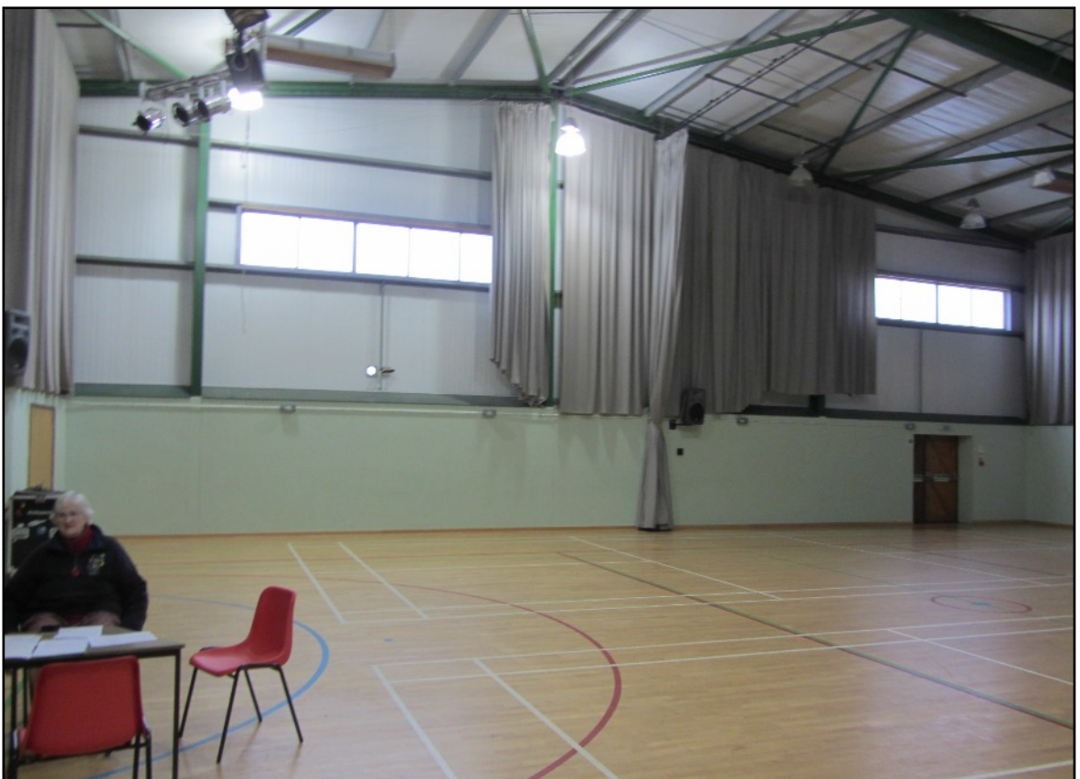
ABOVE The hall is lit by high windows in the east wall. A curtain rail across the ceiling allows the right hand section of the hall to be curtained off. There is no ceiling the hall is open to the roof of a metal framework with cladding which no doubt contains some insulation.
