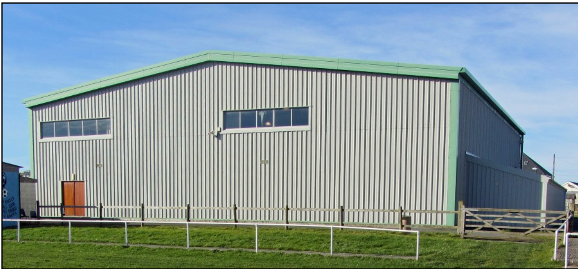
ABOVE The east face of the building. High windows illuminate the large hall. There is one rear door. On the north side is a single storey lean-to.
