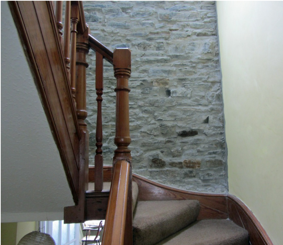
ABOVE On the final flight of stairs some of the wall has been left to show the stonework. . It is interesting that this rubble stone does not include rounded stones from the beach, but this was intended to be plastered and is not 'coursed' carefully like the stone on the front of the villa. BELOW One of the attic rooms, which has a generous head height.
