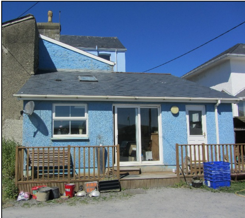
LEFT This is the front which is modern, behind it is a two storey extension on the rear of Carron House.
