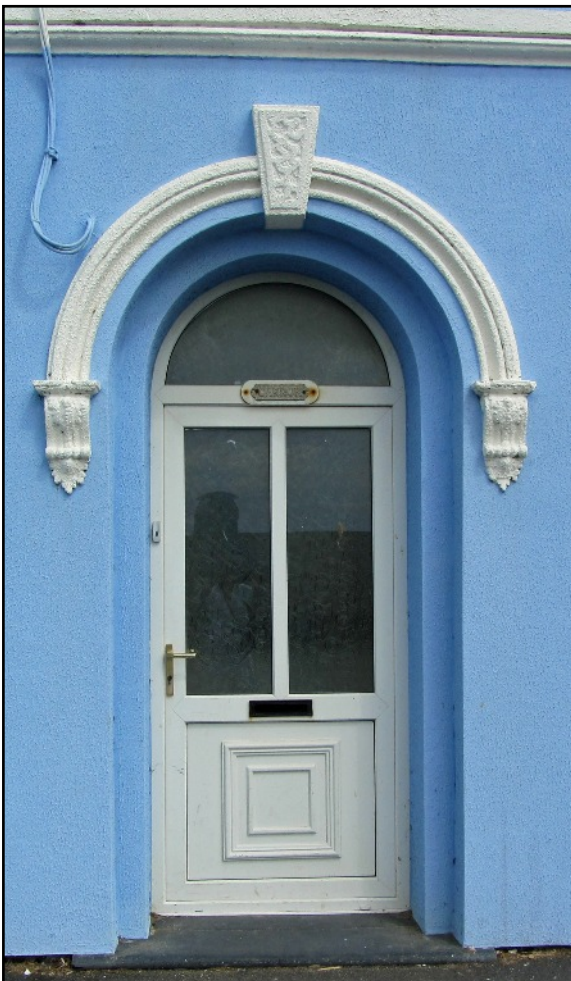
LEFT The front door is under an arch with a keystone, and ends with a bracket each side, its detail now rubbed. A fanlight shaped window above the front door lights the hall. The door is set back making a narrow porch which is some protection from the weather.
