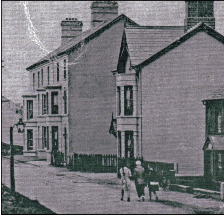
LEFT Carron House had a large brick chimney which we can see in this detail from an old postcard. In the foreground is Maes Arfor (Sea View) then Surrey which had been built in the plot next door we saw on the 1905 map, and beyond is the terrace. The chimneys had five chimney pots (five flues). The chimneys have stripes round them, and locally at this time such chimneys were yellow brick with red stripes. (Postcard private collection - the card had some damage, hence the white mark at the top left.)
