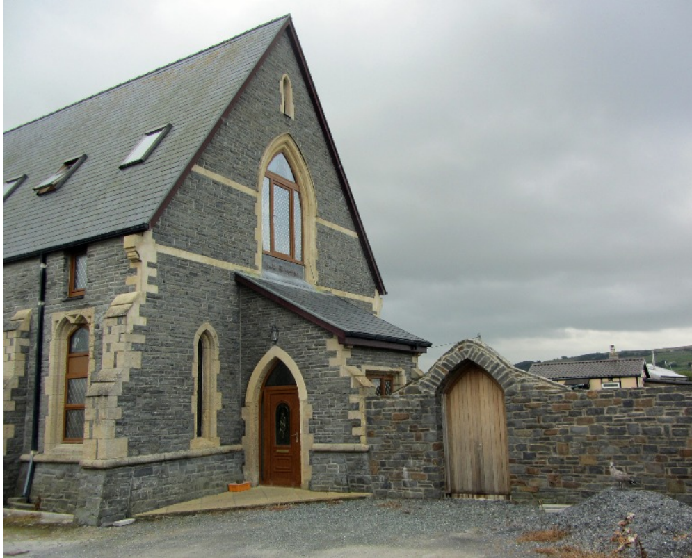
ABOVE The west end, and the entrance to the second home in 2016. The windows and door are modern.
