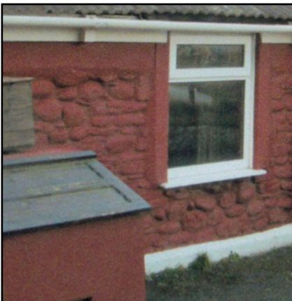
LEFT The walls are rubble stone at the front with plenty of rounded stones from the beach as was usual in Borth's oldest cottages. Mr Peter Matthews of Leronian has said that two of its walls are clom (mud). These would have had a base often knee high of stones.
