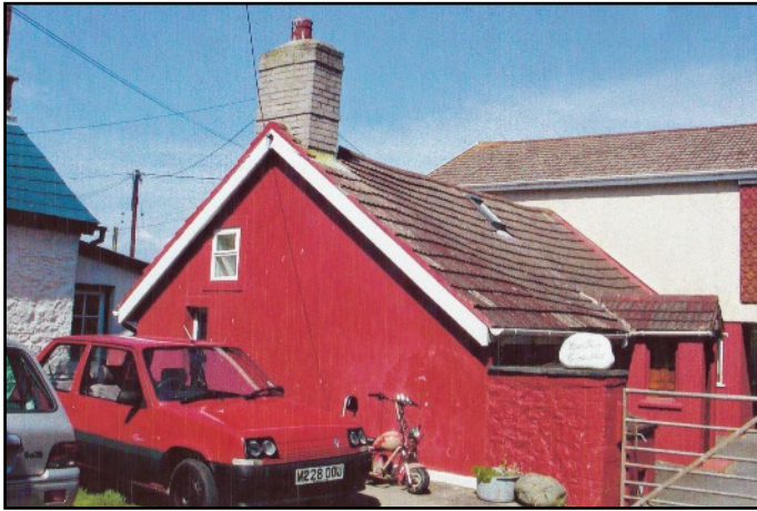
LEFT The west end of the cottage. Its chimney is substantial with sixteen courses of pale coloured bricks.
