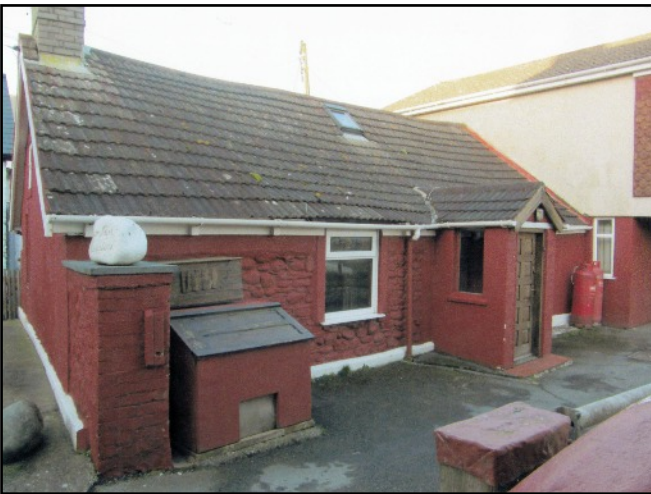
LEFT The old cottage with a chimney on its western end. The front door is not in the centre allowing a larger room
