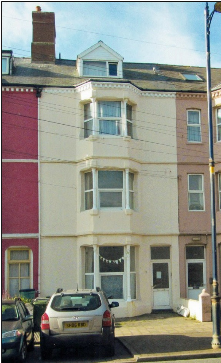
Number 9 in 2014. There were no front garden areas when the houses were first built - they opened directly on to the street, and the dormer window has been added. The house shares a slab brick chimney with Number 8.
