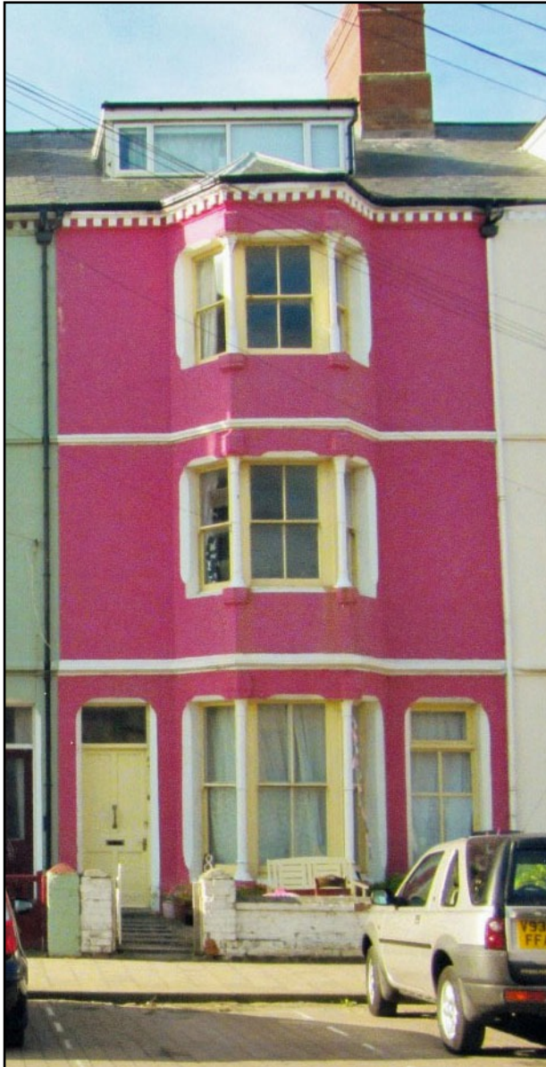
Number 8 in 2014. Like many houses in the Terrace it has a dormer window added in the roof for an attic floor. It shares the slab brick chimney with Number 9.
