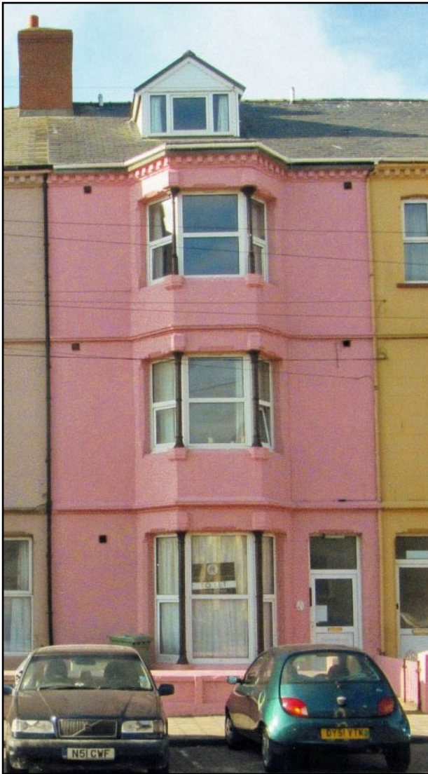
The house in 2014. It shares a slab brick chimney with Number 10. A dormer window in the roof has been added, and there was originally no front garden, the front door opened directly on to the street.
