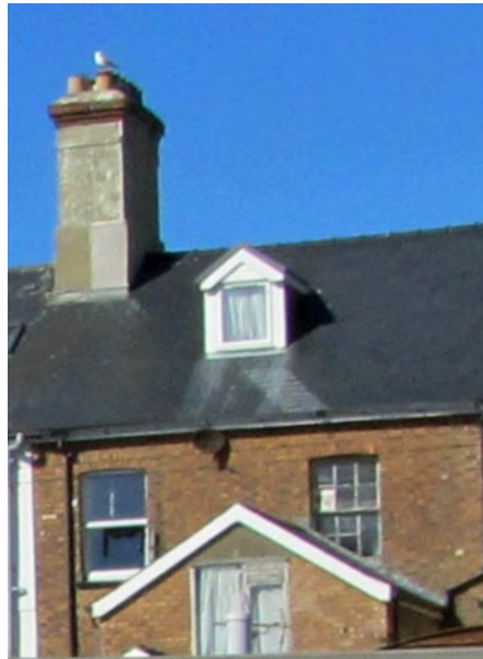
Rear windows at Bibury (Number 2). The photograph on the left was taken in 2009, the one on the right in 2016 when the left hand window had been replaced by a modern one, though keeping the sash pattern. The right hand window is probably an old one. It is likely that all the rear windows of the Terrace were sash windows with twelve lights.
