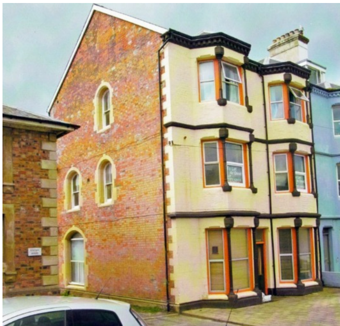
ABOVE Rutland House, Number 1 the Terrace today. The former sash windows have been replaced by modern windows in the same pattern, but the house is open to the street - as all the houses once were. The houses 2 to 10 now have front gardens.
