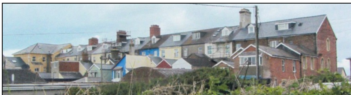
BELOW The rear of the houses in 2014. Four slab chimneys remained.
