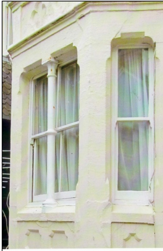
RIGHT This is a window of a house in Queen's road Aberystwyth in 2014 which also has Gothic columns and carved stone dressing beneath its rendering. Gothic columns are also found in Savin's Castle Hotel of 1864/1865 now part of the University.
