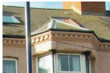
ABOVE The decoration of these houses was enhanced by a pattern made by protruding bricks at the eaves inside a moulded frame. This is Number 10. Each bay was topped by a hipped roof and most of these have survived.
