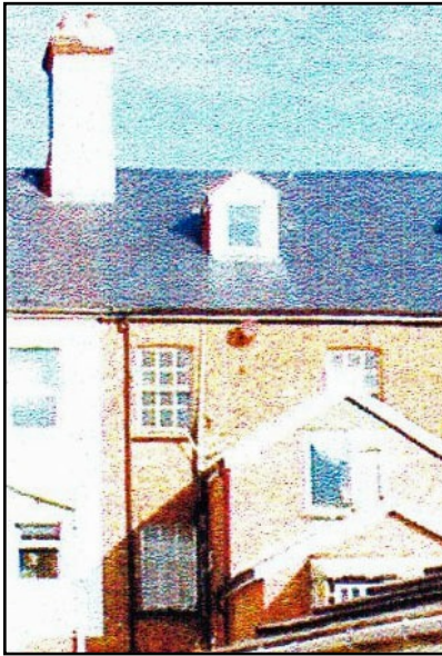
Rear windows at Bibury (Number 2). The photograph on the left was taken in 2009, the one on the right in 2016 when the left hand window had been replaced by a modern one, though keeping the sash pattern. The right hand window is probably an old one. It is likely that all the rear windows of the Terrace were sash windows with twelve lights.
