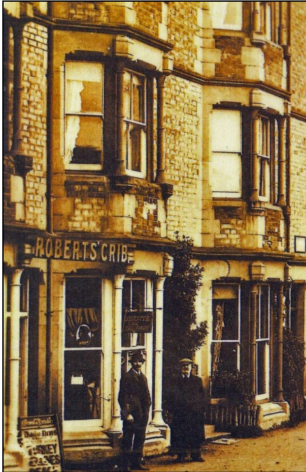
LEFT Robert's Crib, the shop in the foreground was in Number 1, Rutland House, in 1924. The first four houses in the row still had their bricks showing, and the sandstone dressings were quite bold and decorative (Detail from a postcard by courtesy of the Amgueddfa Ceredigion Museum).
