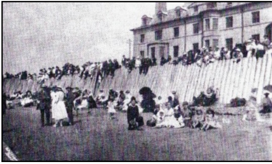
LEFT A postcard by Williams of Borth shows the wall of planks anchored into the bank to protect the Esplanade and the Hotel from the sea. The beach was then sand and not stones as today (Courtesy of the County Council)
