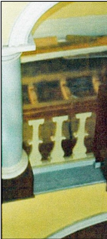
ABOVE The banisters appear to be flat cut-out shapes. Behind are pieces from dismantling the building.
