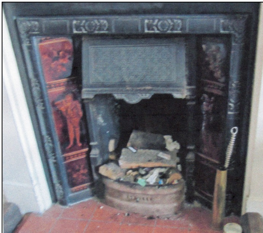
LEFT This fireplace is in the living room on the south side of Caerffynnon.
