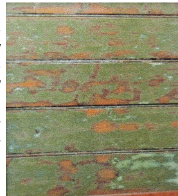
RIGHT The house has panelled walls. This detail which has been saved shows the old painted surface.
