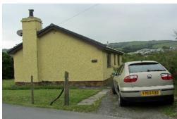
The bungalow is built on a platform on flat land reclaimed from the Cors Fochno between a footpath and an old watercourse, now a deep ditch. It has a brick base, and the remaining walls are rendered. There is a chimney allowing a fire or stove in the lounge.
