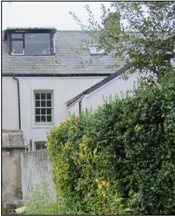
ABOVE The rear of Bushbury in 2015.
