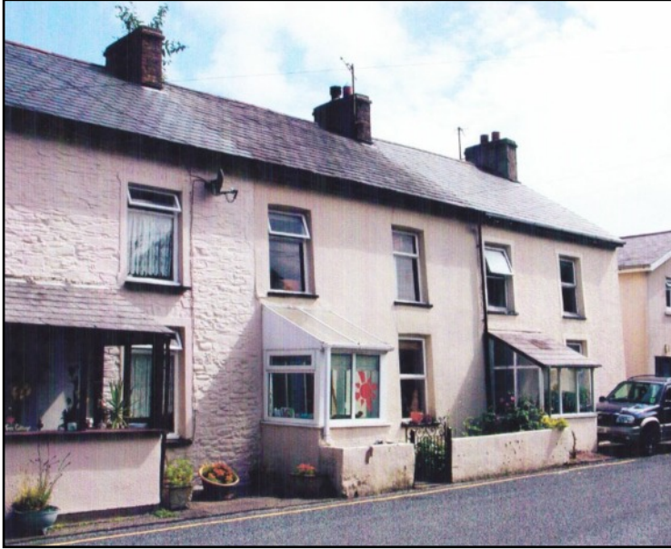
ABOVE The Terrace in 2009. Bushbury is in the centre.
