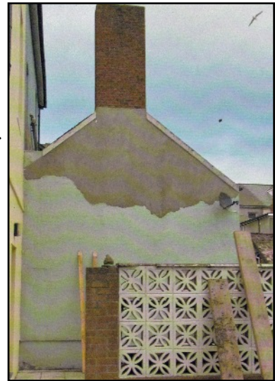
LEFT The entrance passage to the cottage past Bronheulyn House showing the beach pebbles in the wall from the old cottage. This cottage had an upper floor and stairs, and the beach pebbles go right up to the top of the gables. These walls would have had lime plaster and coats of lime wash to protect them, and though dampened by rain, would dry out and keep the inside of the cottage warm and dry.
