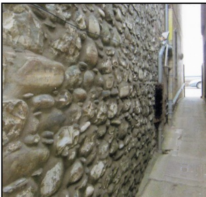
LEFT The entrance passage to the cottage past Bronheulyn House showing the beach pebbles in the wall from the old cottage. This cottage had an upper floor and stairs, and the beach pebbles go right up to the top of the gables. These walls would have had lime plaster and coats of lime wash to protect them, and though dampened by rain, would dry out and keep the inside of the cottage warm and dry.
