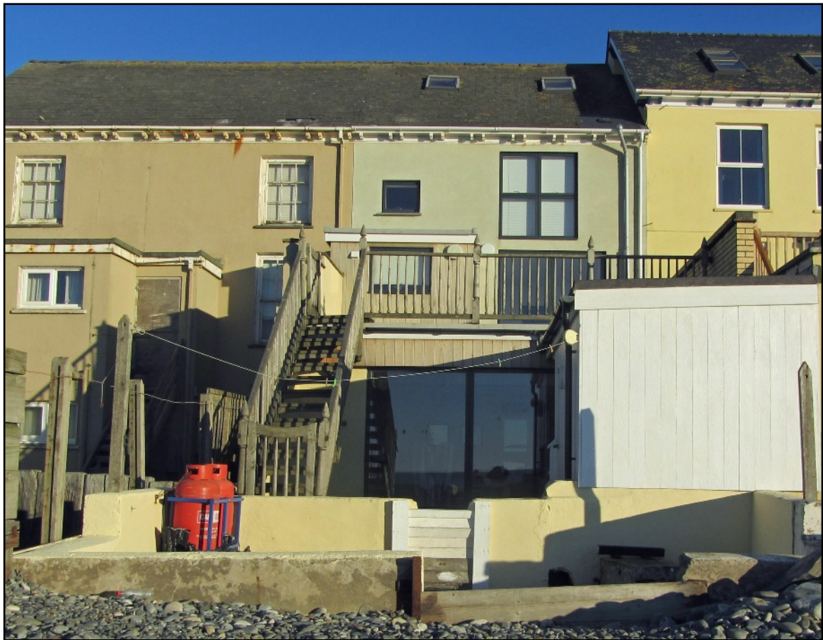
The rear of the house from the beach in 2016.
