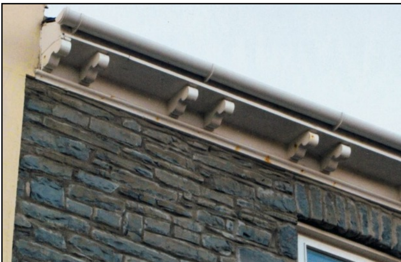
LEFT These are the brackets (dentils) supporting the overhang of the roof. They were commonly used for the buildings in this terrace. Tops of the windows like this, probably stone, are on the older houses and cottages in Morfa Borth. The stones of the wall are coursed but vary very much in size and shape. Photo taken in 2015. The rendering had been removed.
