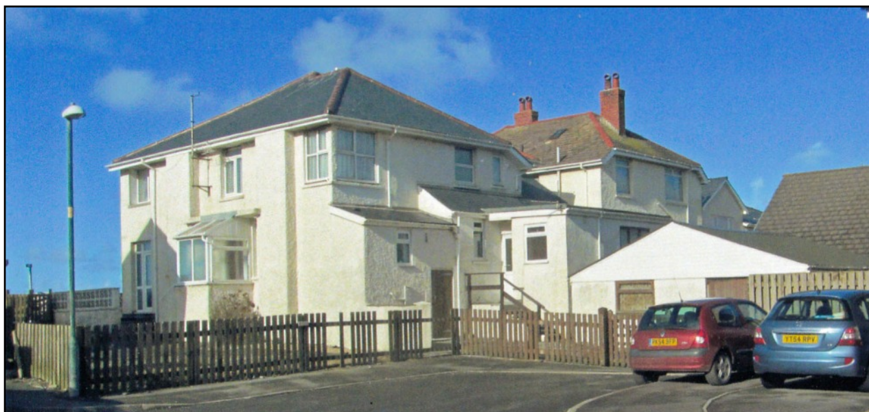
ABOVE The rear of Benfleet in 2016
