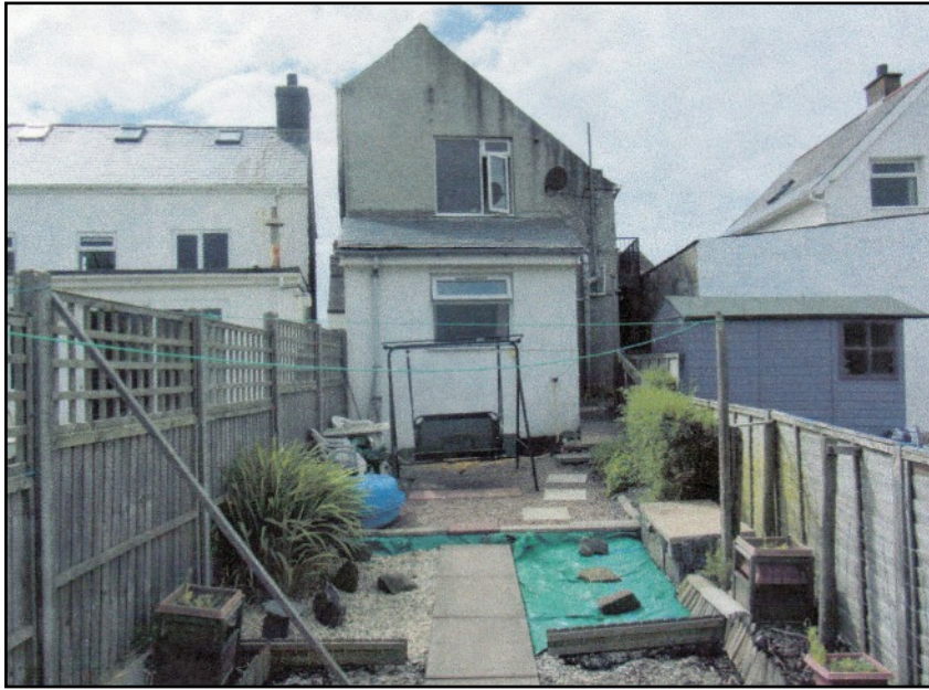
LEFT The rear of the house, with a different shaped roof from the front section, and with a single storey lean to extension as well. There will be a good view from the upper window across the railway and pastures to the hills. The garden belongs with the lower flat. It faces east and it becomes long and narrow extending to the ditch which was once a brook with fresh water for the old cottages.
