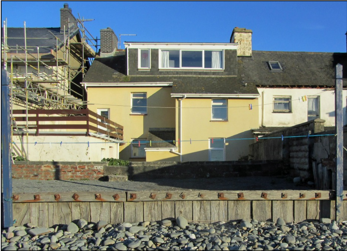
The rear of the house from the beach in 2016. A large dormer window gives a good view of the sea. The extension on the south side of the yard was already there in 1886. The building on the north side has a balcony for good views of the beach. A tall wall encloses the north side of the yard. All the rear windows are modern.
