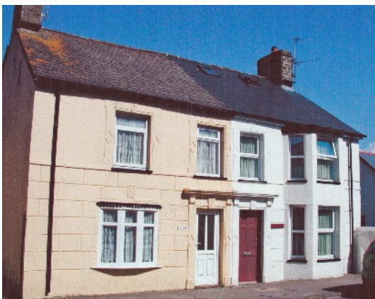
LEFT Alma on the east side of the High Street is one of a pair with Glanaber.
